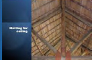
Roof Interior - Bamboo cross timbers and rope lashing
